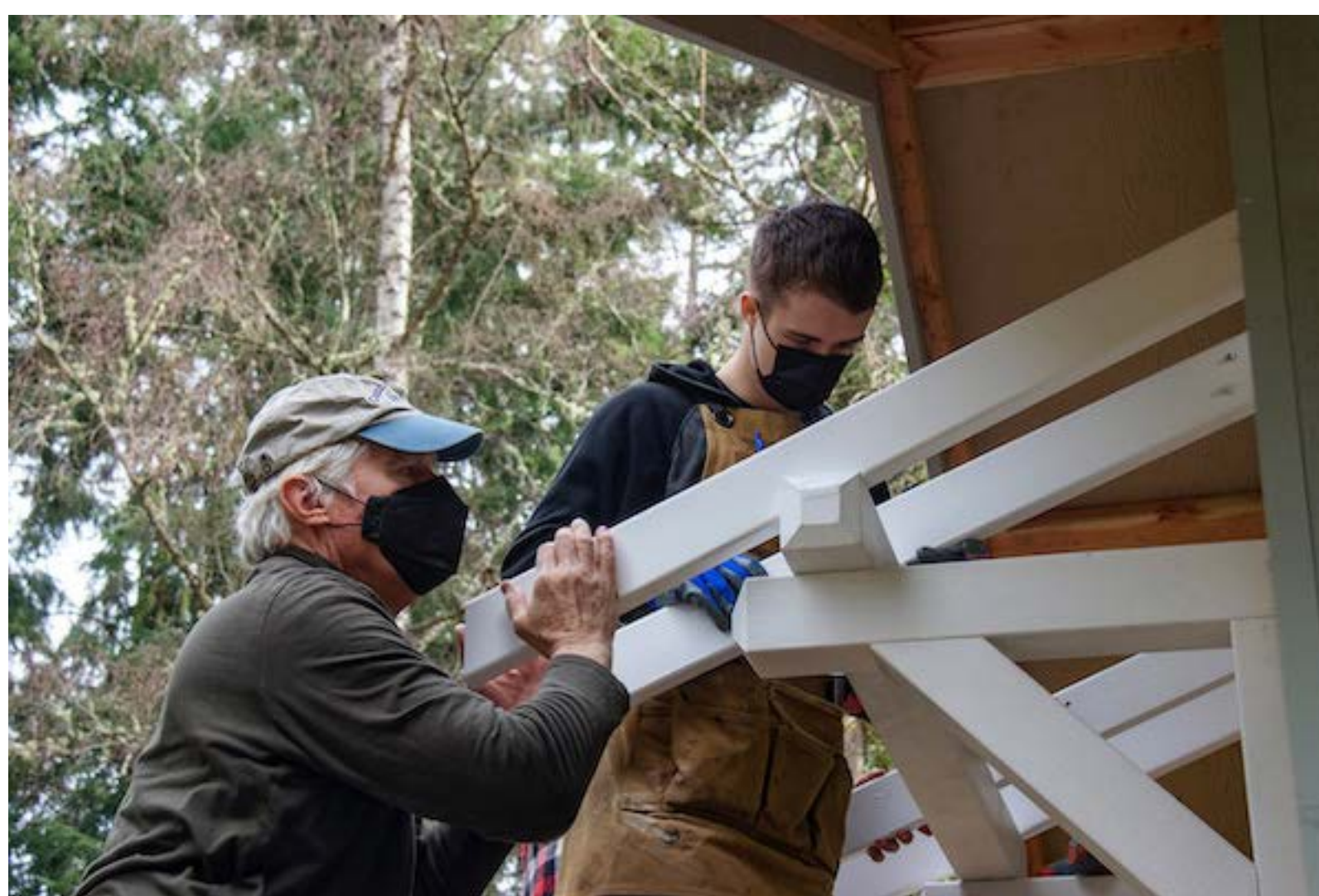
Joe working with a Woodhaven student to add a portico to the tiny house.
